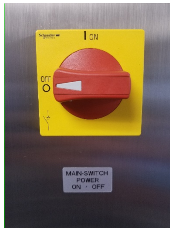
Figure 3 - ICU main power disconnect switch
