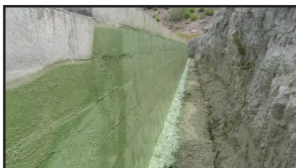
READY FOR BACKFILL
