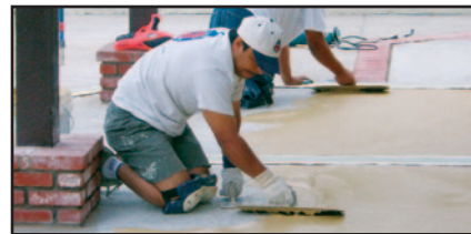
BASE COAT APPLICATION – TROWELED
