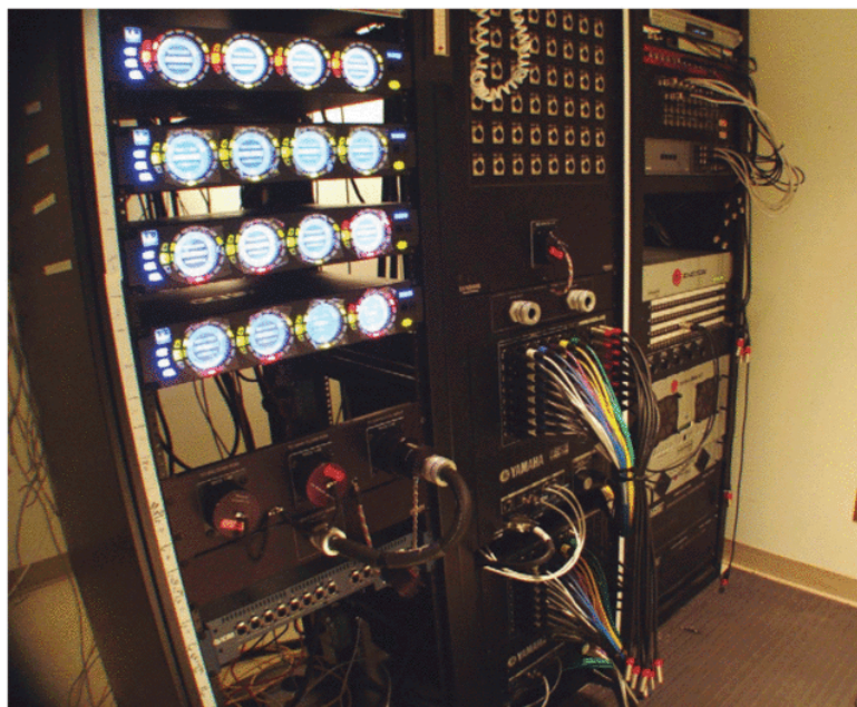
These equipment racks house Dolby Lake processors, Yamaha digital input boxes and Whirlwind E Desk and E Snake devices.
