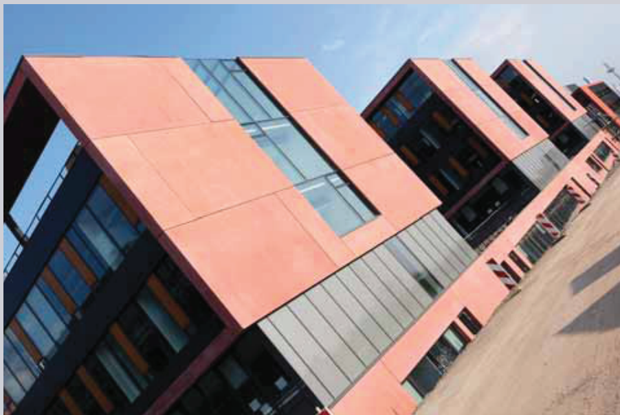
Campus Riedberg of the Gothe University in Germany completely networked using Dante
